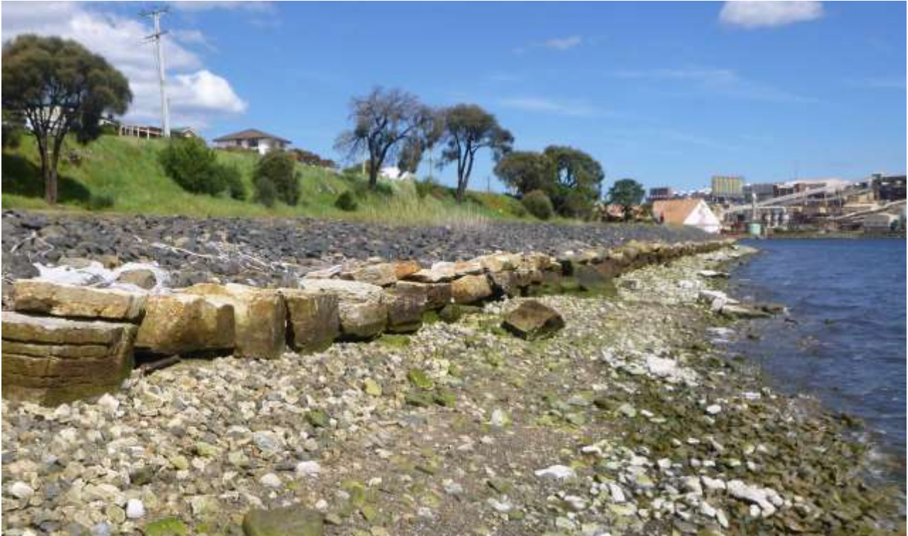
Figure 23: New seawall constructed circa 2020 at East Risdon, Derwent Estuary. This robust boulder wall protects a shore at Saunderson's Road (East Risdon), which was previously exhibiting significant erosion in the cobble-grade artificial fill visible above and below the new boulder wall. This material was previously directly exposed to the wake waves generated by the Mona Roma ferries which pass through this narrow reach of the Derwent Estuary several times a day. Photo by C. Sharples (21 st October 2021).
