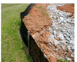
**Sediment controls** capture soil that is already eroding and prevent it from leaving your site.
