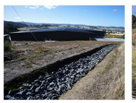
**Drainage controls** divert upslope runoff around your site, reducing the amount of water needing to be treated.
