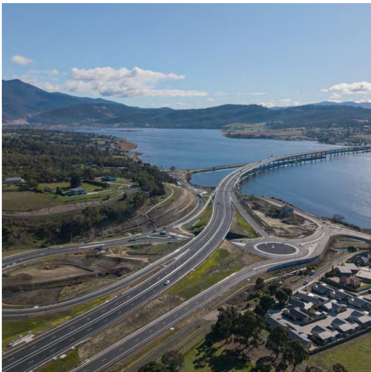
Figure 5.6 New Bridgewater Bridge Project – Image provided by the Department of State Growth 2025 – https://www.bridgewaterbridge.tas.gov.au/current_work/images_and_video
