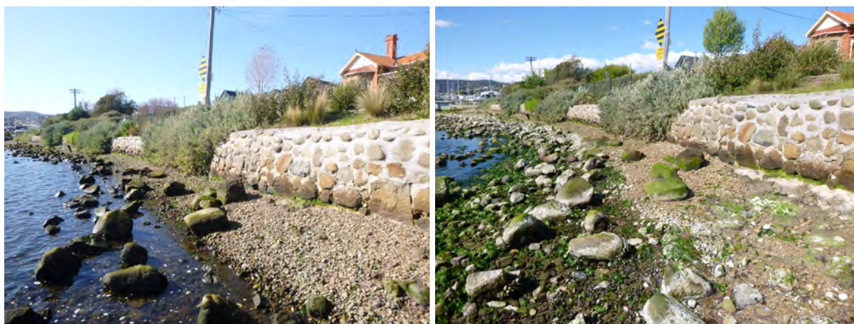
Figure 9.19 Comparison of KBPP5 monitoring photos captured on 08/08/2021 (prior to ferry operation) (left) and 21/10/2021 (right). Left image shows a cobble-dominant foreshore, and right image shows more exposed underlying dolerite bedrock, particularly towards to lower right-hand area of the photo. Image: Chris Sharples.
