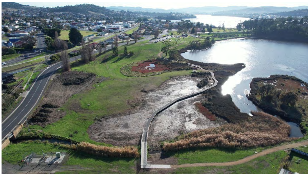
Figure 9.17 Aerial imagery of Windermere Bay saltmarsh restoration site after Stage 2 excavation works were complete. Image: Mark Bachmann, NGT.
