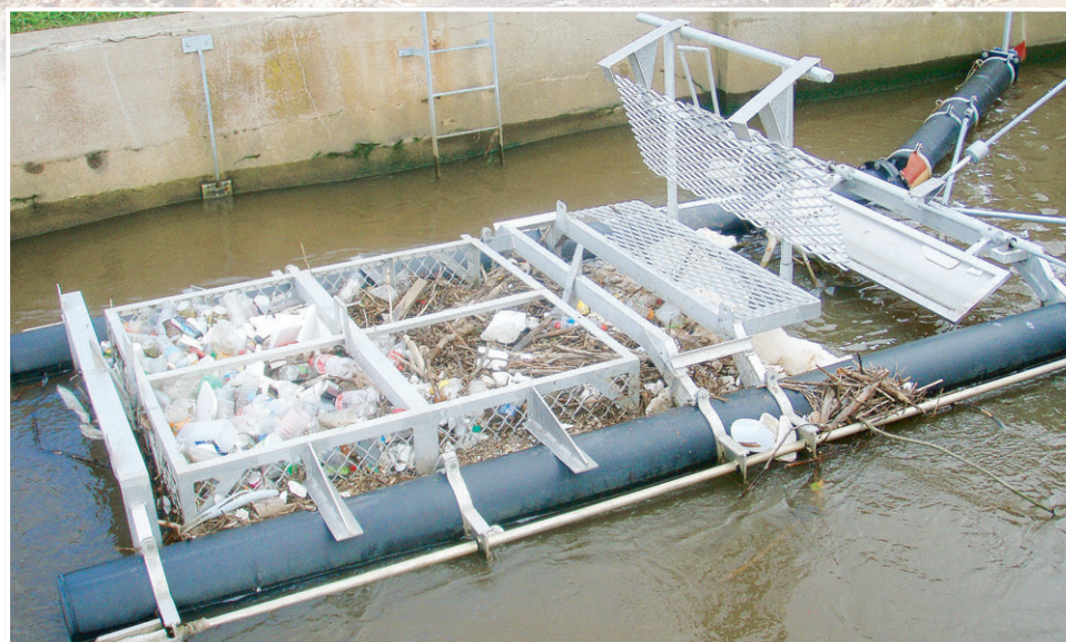
ABOVE: Litter traps are used to prevent litter from entering the Derwent.
