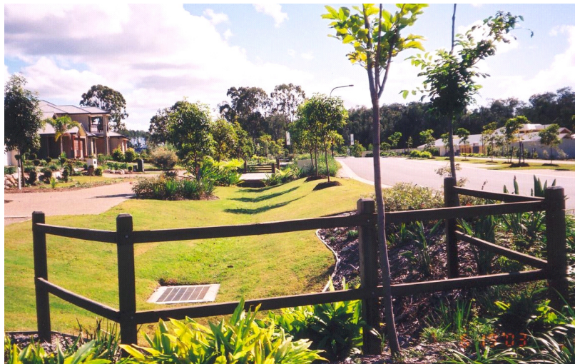
Figure 0.12. Photograph of bioretention swale
