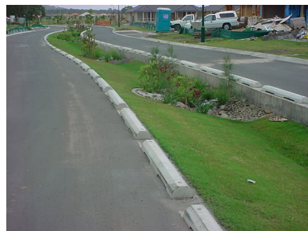
Bioretention swales are commonly located in median strips of roads and carparks
