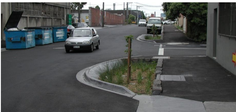
Figure 5.7. Retrofitted Bioretention System in a street
