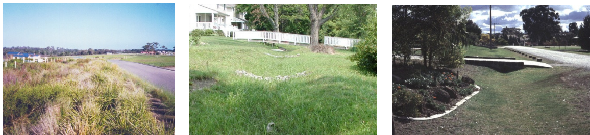
Figure 0.2. Swale systems: heavily vegetated, use of check dams, grass swale with elevated crossings
