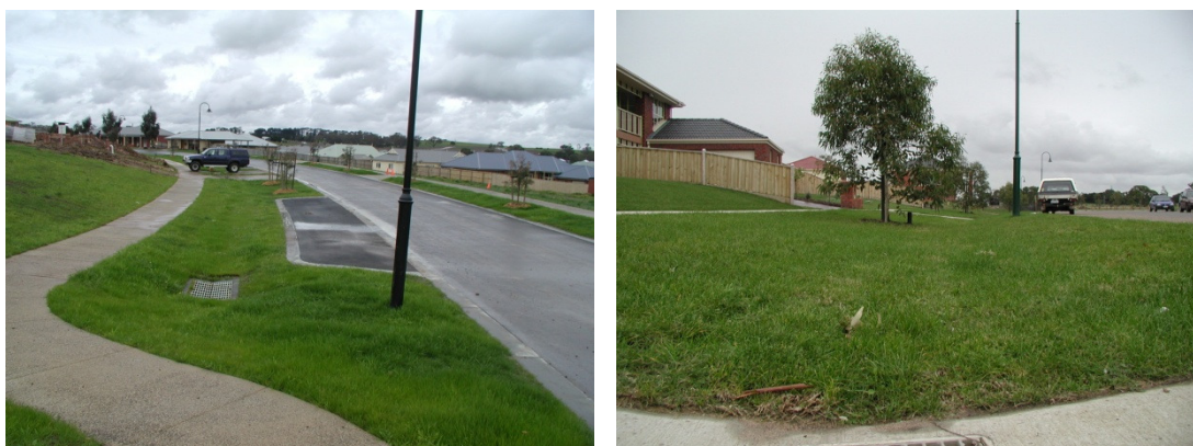
Figure 0.17. Similar buffer swale system for conveying runoff
