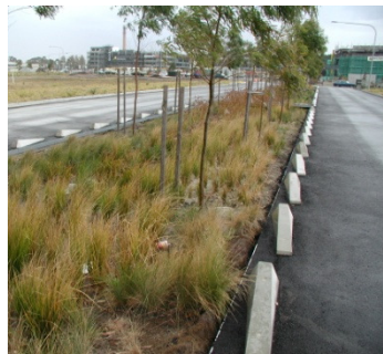
Figure 0.12. Photograph of different arrangements of kerbs with breaks to distribute inflows
