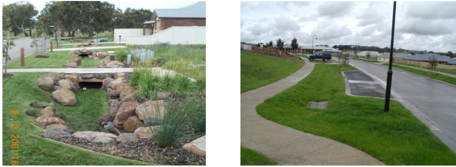
Figure 0.3. Elevated and at-grade driveway crossings across swales
