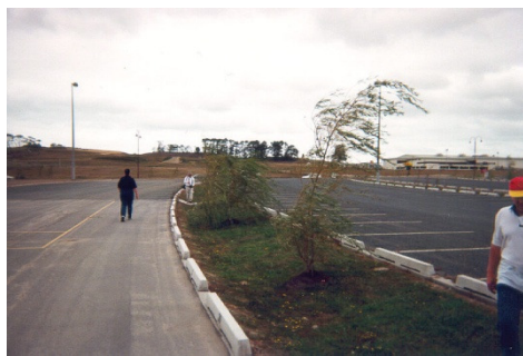
Figure 0.12. Photograph of different arrangements of kerbs with breaks to distribute inflows
