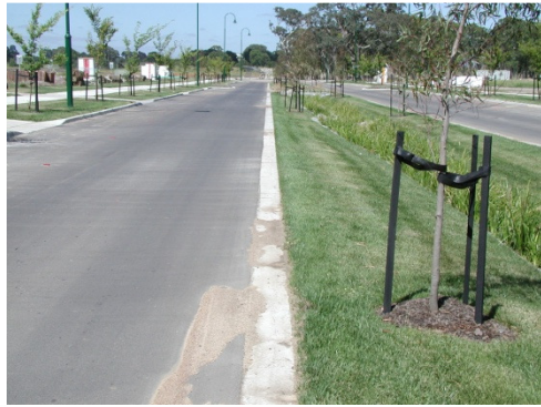
Figure 0.11. Photograph of flush kerb without setdown, edge detail showing setdown
