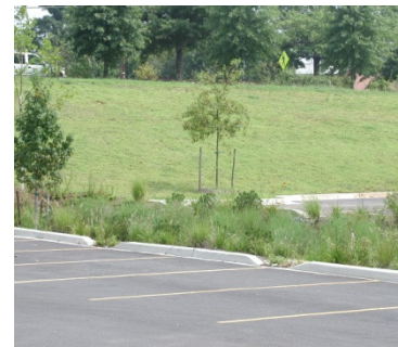
Figure 0.12. Photograph of different arrangements of kerbs with breaks to distribute inflows
