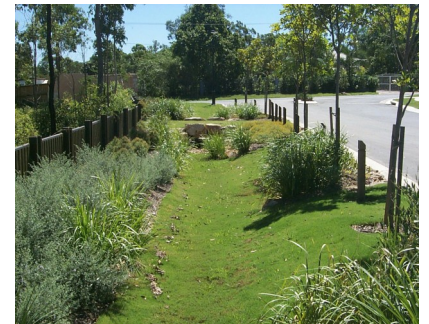
Figure. Example of a vegetated swale (instead of a drain)
